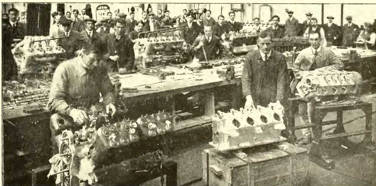
A BRITISH AERO-ENGINE SHOP.—The erecting shop of the Sunbeam Works, which is now turning out quantities of high-powered Sunbeam engines to Mr. Louis Coatalen's designs, for seaplanes.
